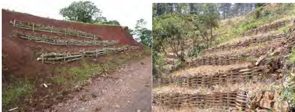
Figure 14: Bio-Engineering Works
